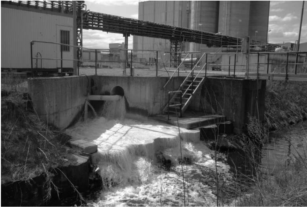
Figure 2: The industrial wastewaters are disposed of in the Eindergatloop. Although the content of heavy metals is currently being monitored, a recent report revealed that the contaminants levels are still dangerously high (Vlaamse Milieumaatschappij, 2018).
