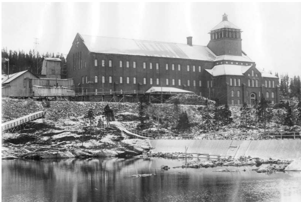
C. The switchgear building in Bårjås around the time of the inauguration.
